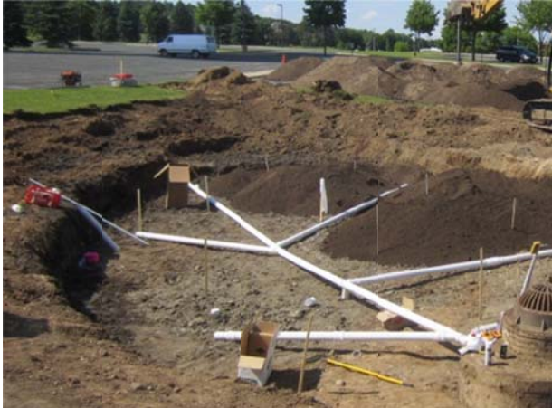
Installed underdrain and backfilling with engineered soils
