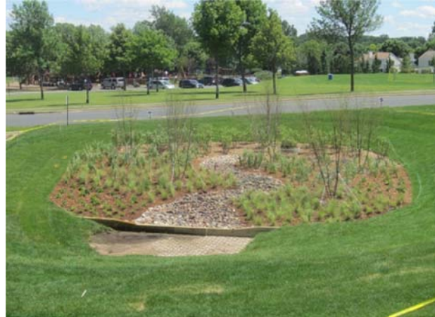
Installed dry creekbed, mulch, trees, shrubs, grasses, and flowers
