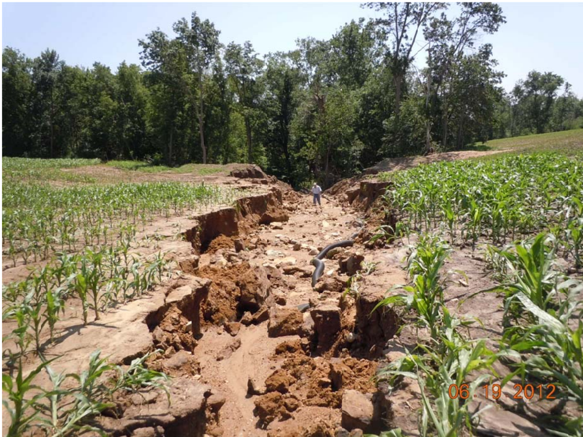
Example of Flood Damage from June 2012 – Douglas Township
