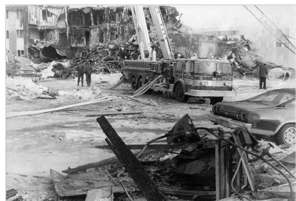
Figure 4.18 Propane Explosion and Fire, West St. Paul, 1974
