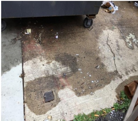
Enclosure MPL32 – broken glass inside enclosure
