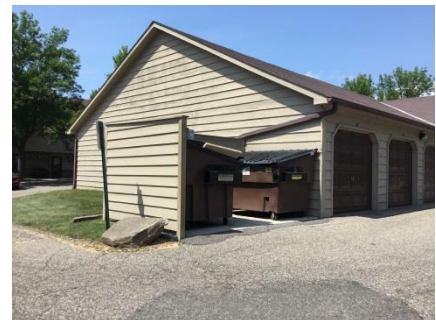
Enclosure CHK7 – no recycling provided
