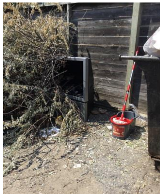
Enclosure CHK3 – yard waste inside enclosure
