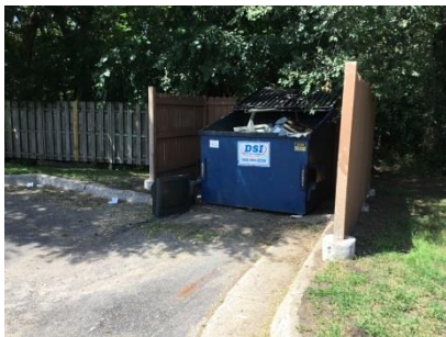
Enclosure CHK2 – no recycling provided
