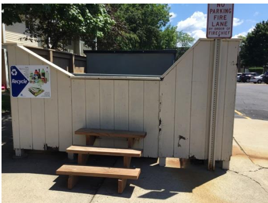
Example of adequate signage on exterior of enclosure
