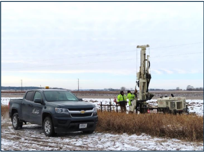
Environmental Well Installation, Hampton Township, January 2022
