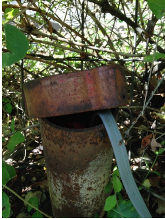
Figure 5: Coliform bacteria-positive well lacking watertight and vermin-proof cap/cover
