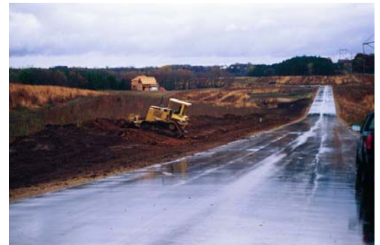
Large lot development above the ravine would impact the ecological and aesthetic value of the park.
