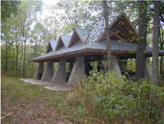
One of two existing picnic shelters tucked into the woods
