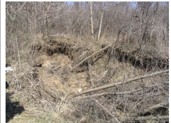
Gullies are forming within the ravine because of heavy runoff volumes from the fields above the park.
