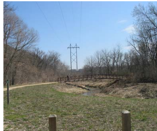
Trout Brook Bridge
