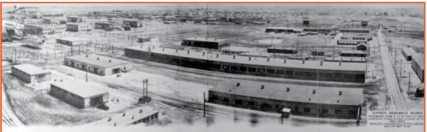
View of the Gopher Ordnance Works in the mid 1940s. Source: Dakota County Historical Society
