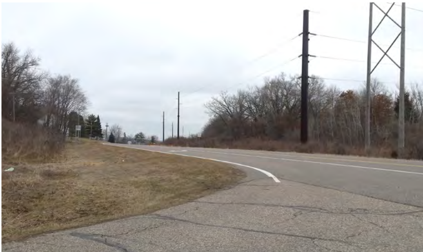
Looking from the St. Thomas Becket parking lot to the east, the Highline corridor crossing of TH3 / S. Robert Trail sets up topographically well for a bridge, but the numerous power poles and lines provide a challenge to work around.
