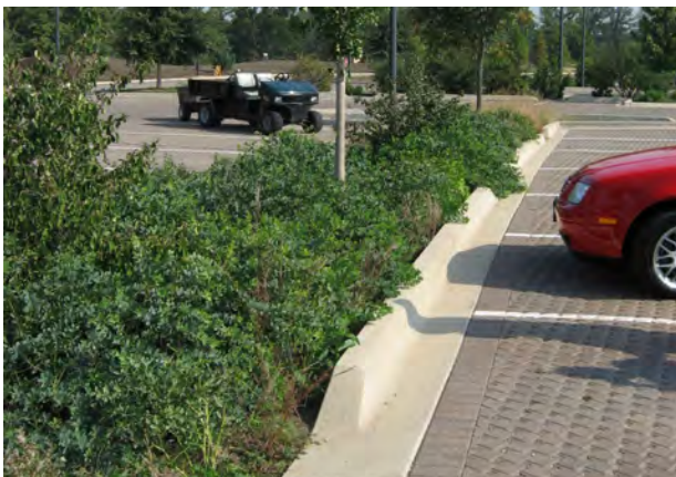
Pervious pavement and rain garden in a parking lot
