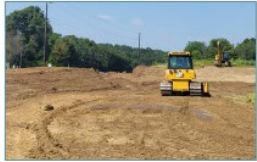
Construction of a water and sediment control basin in Eagan
