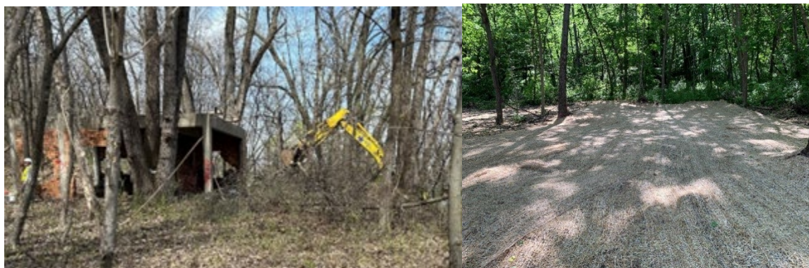
Figure 1. Pump house and well before (left) and after (right) demolition and sealing.
