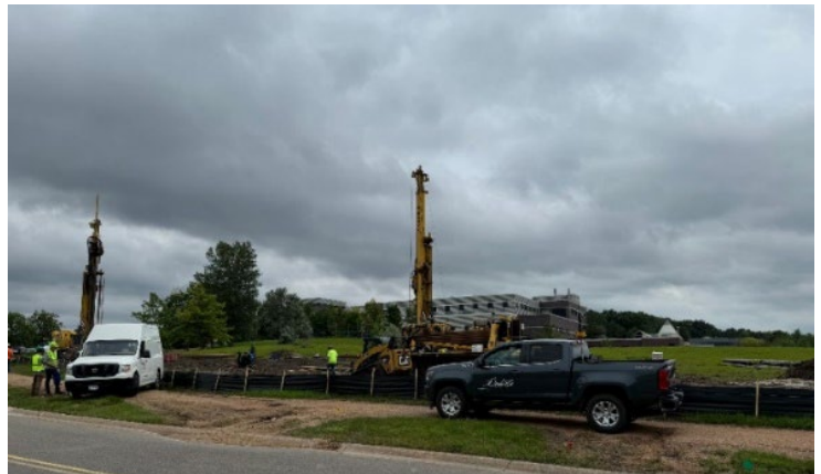
Figure 8. Well construction drill site
