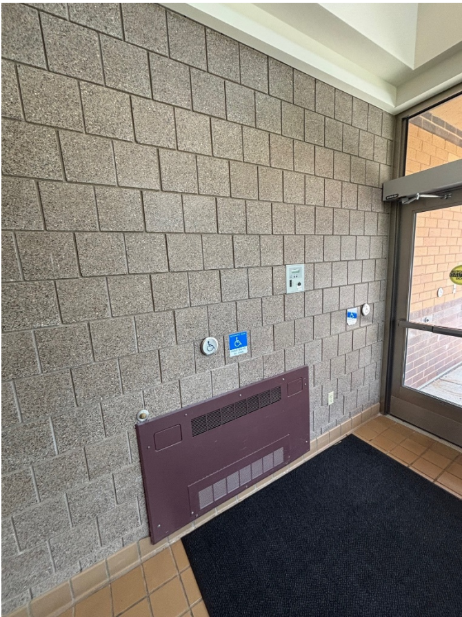
Figure 4 - Fire Annunciator
