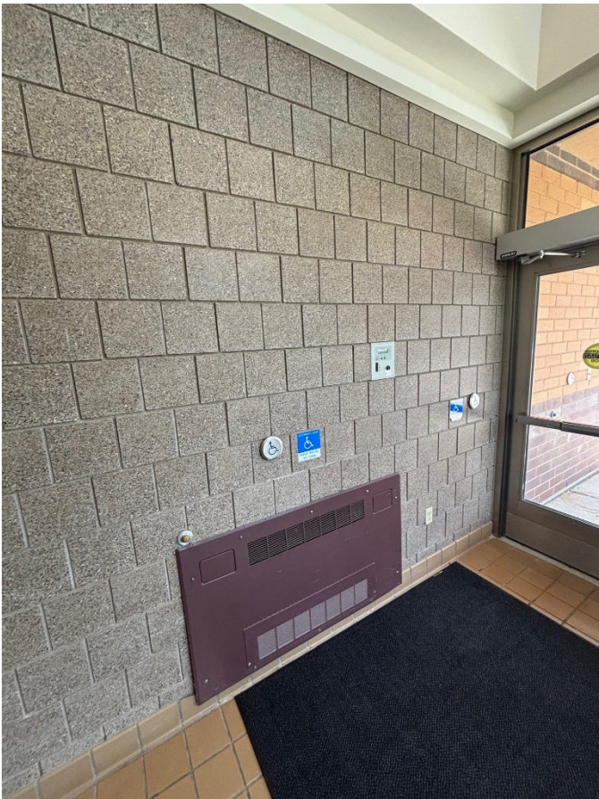
Figure 4 - Fire Annunciator
