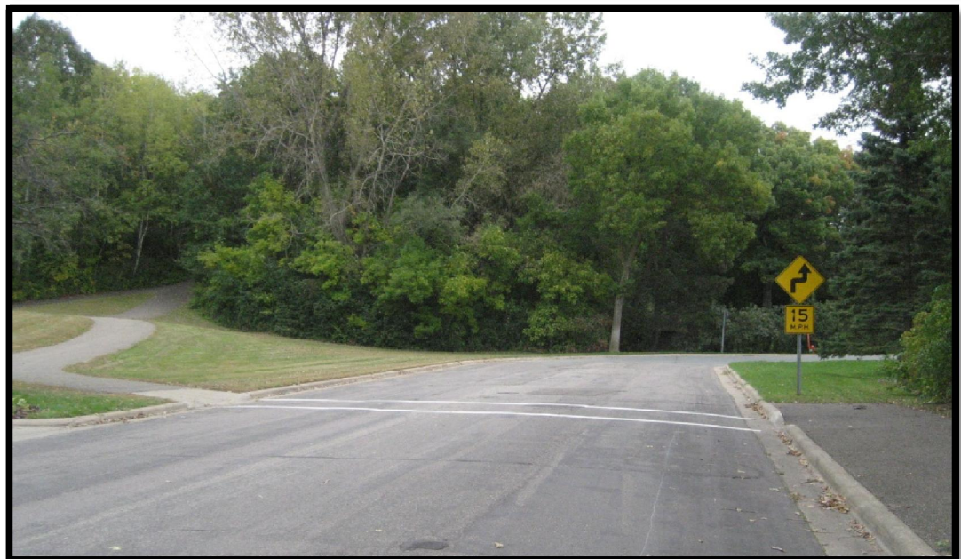
Existing advance signing for the trail crossing on Kraft Road (top photo). Marked crosswalk at the trail crossing, but with no signing (bottom photo).
