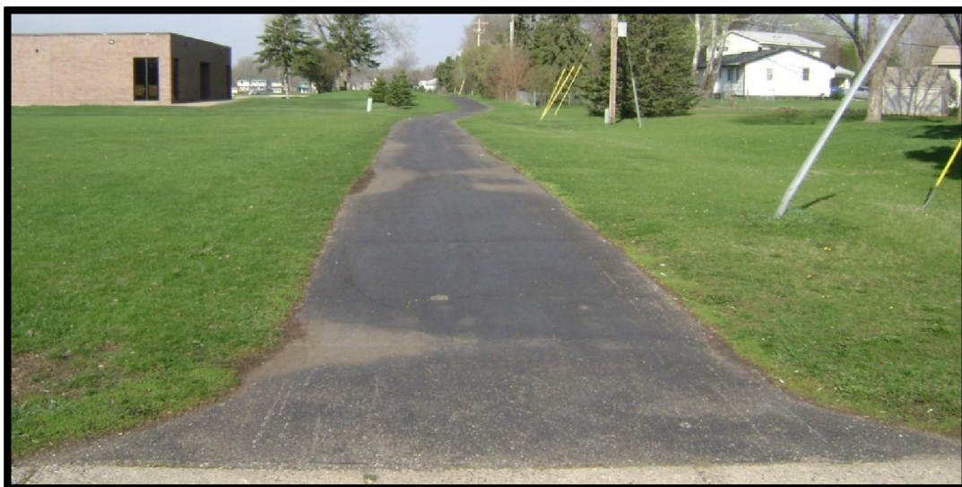
View of the trail running from Foliage Avenue on the north side of the school. There are currently no crosswalk markings or pedestrian ramps to cross Foliage Avenue at this location.
