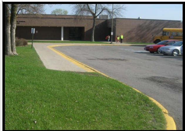
The sidewalk does not extend to the end of the vehicle or bus loading/unloading areas.
