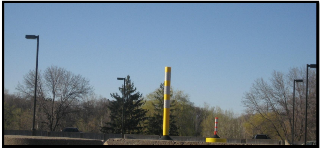
Example of a flexible post delineator.
