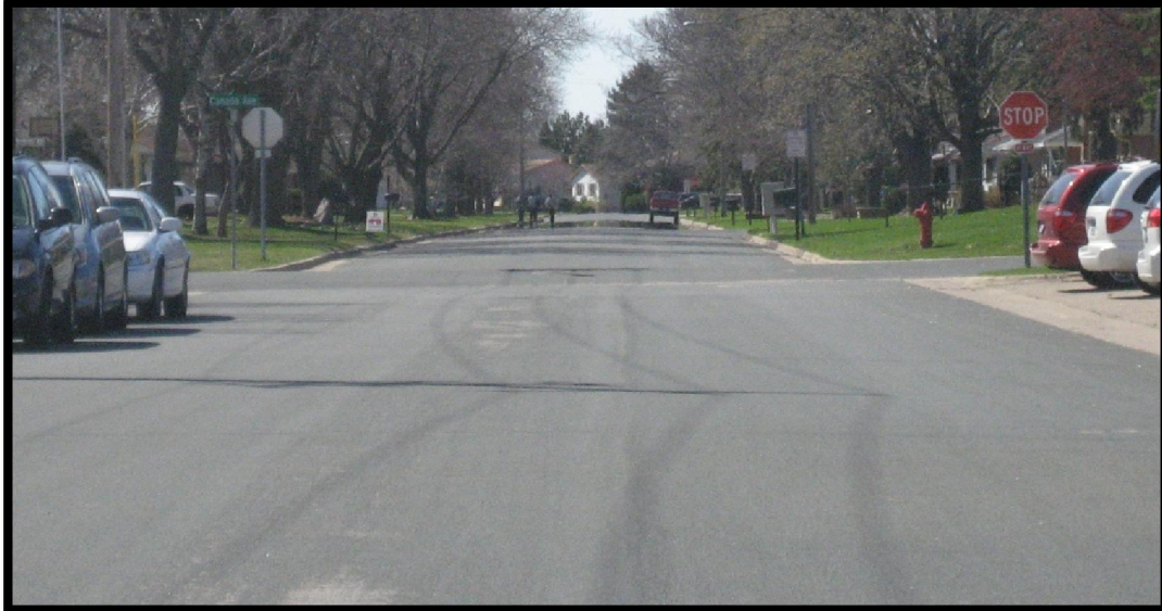
View of 144 th Street looking west from the Rosemount Elementary. There is no sidewalk on 144 th Street west of Canada Avenue.
