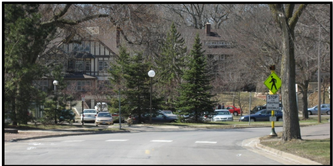
Example of midblock zebra crosswalk with pedestrian-activated flashers.
