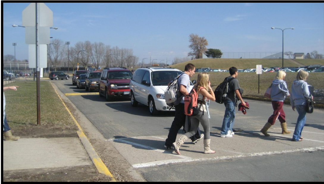
Students crossing traffic flow entering and exiting the parking lot after dismissal. The crosswalk striping is not very visible and there are no pedestrian ramps for the crossing.
