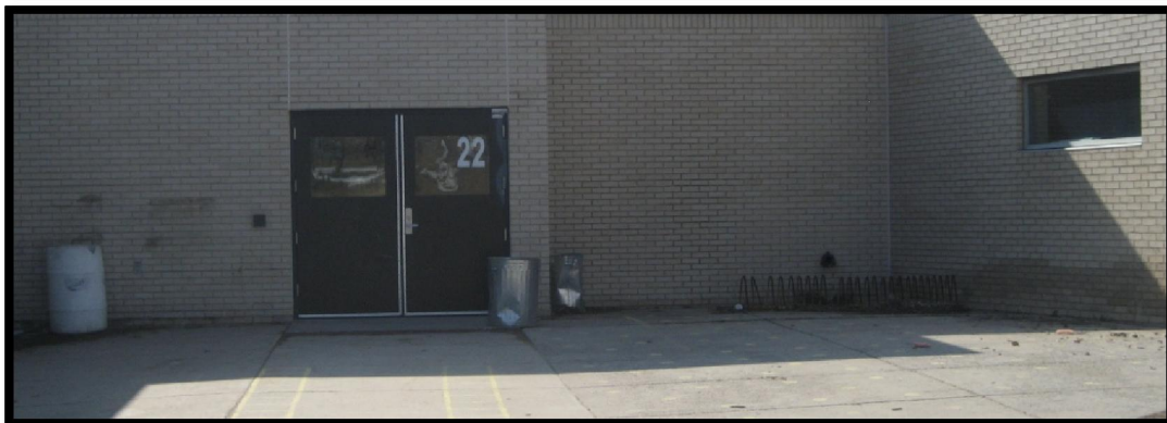
Bike racks located along 142 nd Street (top photo) and next to a side entrance (bottom photo).
