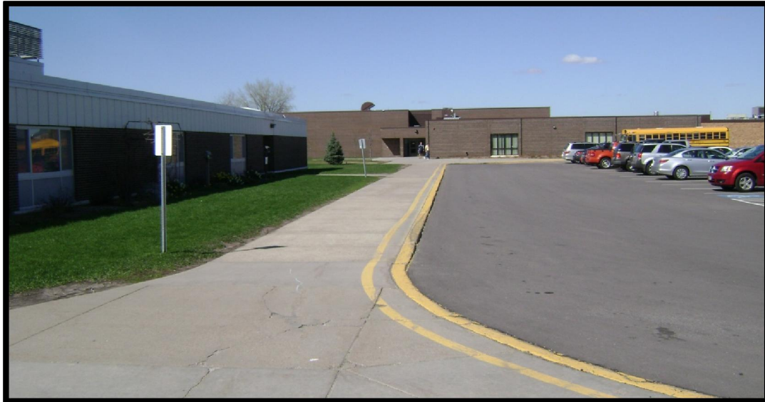
Rosemount Elementary School (left) and Rosemount Middle School (center) share a parking lot for staff and parent parking, as well as bus loading/unloading.
