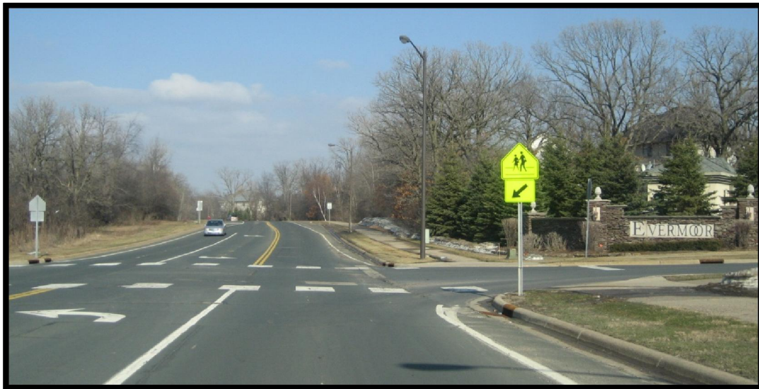
Existing school crossing on Shannon Parkway at Evermoor Parkway.
