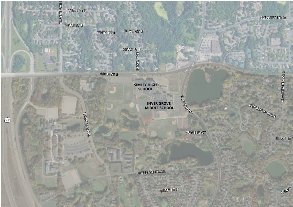
Inver Grove Heights Middle and Simley High School campus and surrounding area
