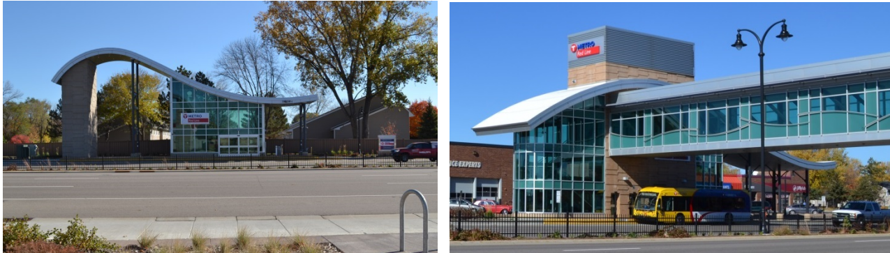
Figure 5. Online Stations, METRO Red Line 147 th Street Station and Apple Valley Transit Station in Apple Valley, MN
