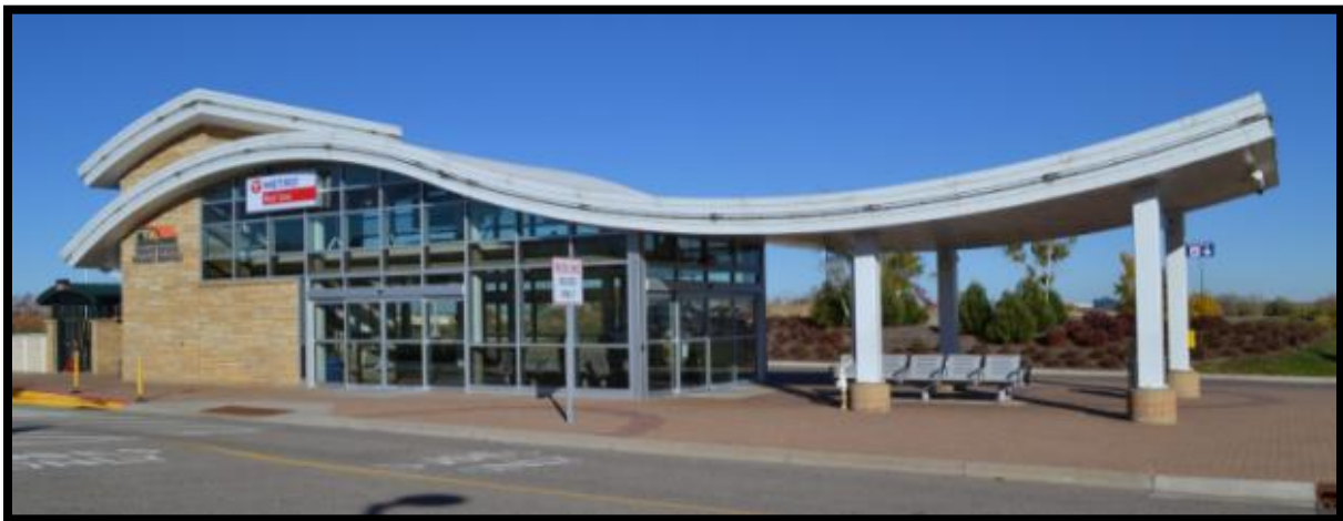
Figure 10. Cedar Grove Transit Station
