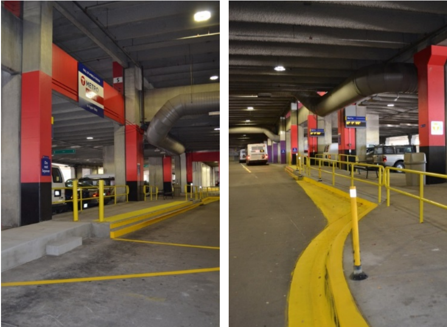
Figure 8. Photographs of the current temporary METRO Red Line Platform
