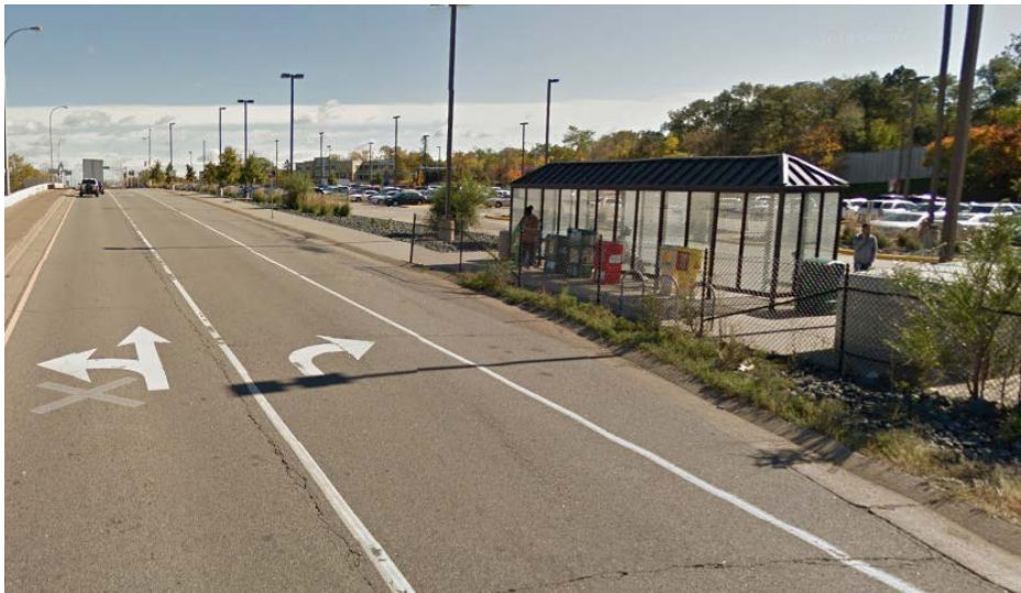
Figure 6. Inline Station, Louisiana Avenue Transit Center in Saint Louis Park, MN
