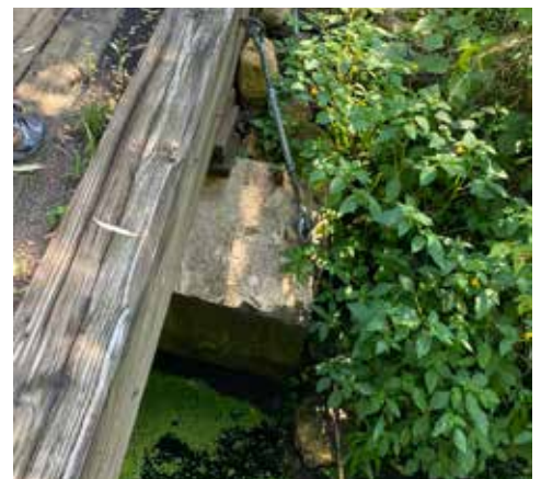
Trout Brook footbridge damage
