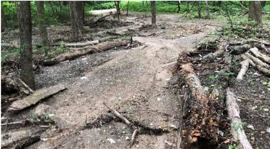
*Eroded gravel and soil from Hilary Path deposited in the forest near existing DNR boat landing*
