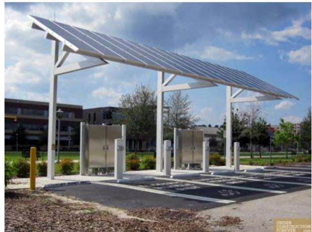
**Photo 57: Example of Electric Vehicle Charging Station with Photo Voltaic Solar Panels**
