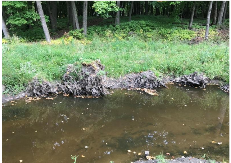
Installed rootwads two years after vegetation establishment and maintenance. The rootwads have grown into the stream bank. Log toe was installed, but is not visible (submerged under the water line) in this photo.
