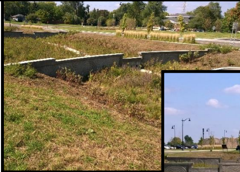
"Stepped" infiltration basin in Oakdale, MN.
