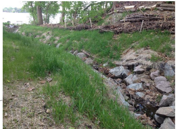
Detail of Vegetated Riprap and photo of installed practice on channel project one year after construction.
