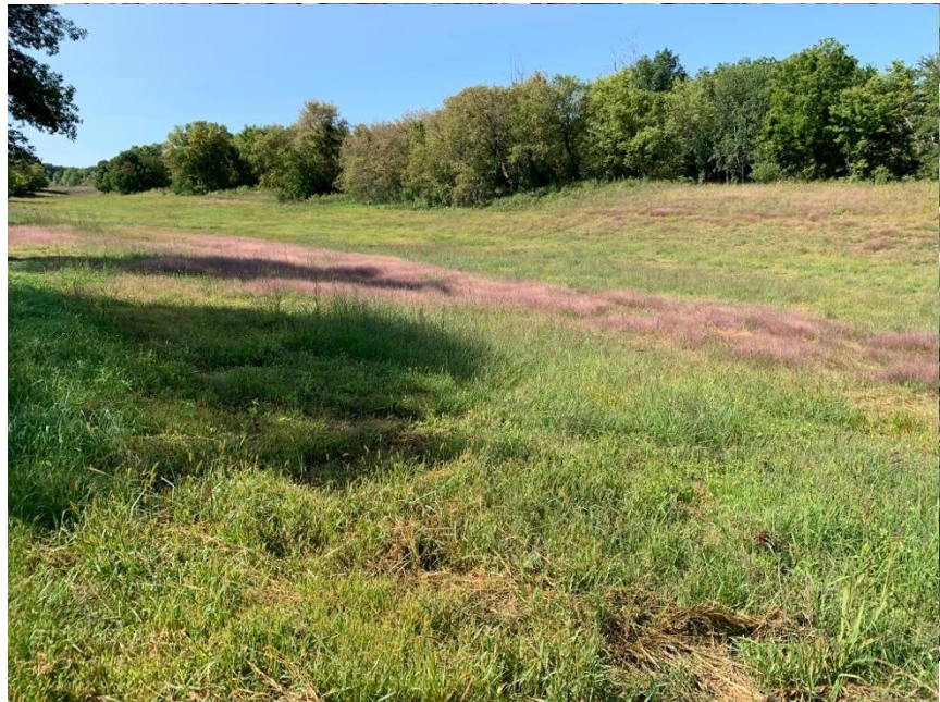
Photo 7. Spillway at Vermillion River Linear Park
