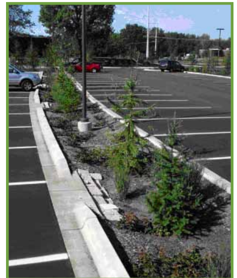
Depressed parking lot islands capture stormwater and water trees that eventually will shade the lot.
