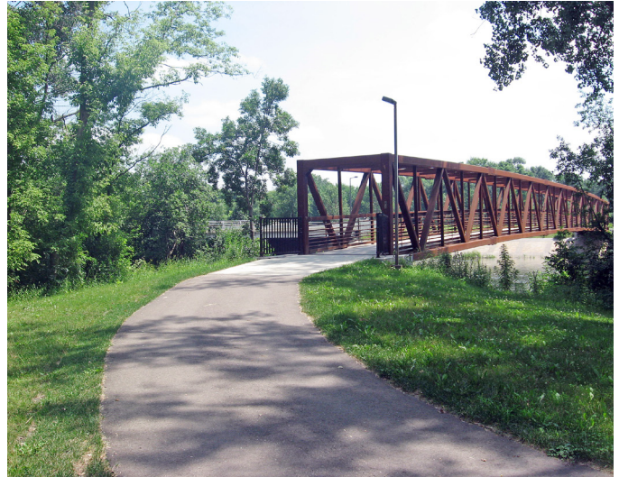
The Mill Towns Trail and Bridge – City of Northfield, Minn.
