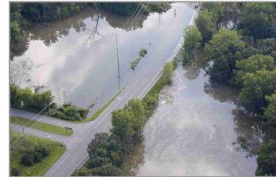
Flooding at Lebanon Hills
