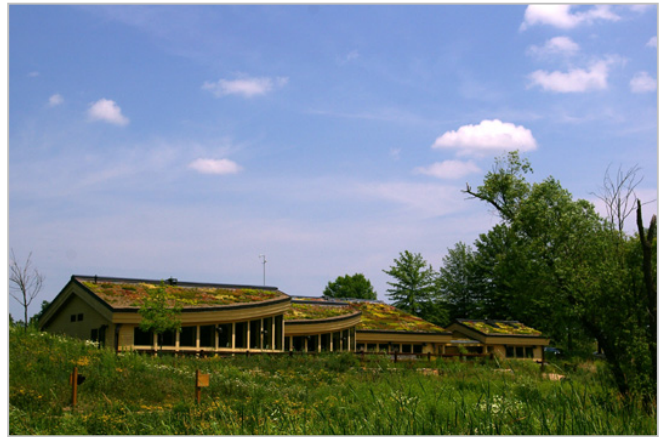
Lebanon Hills Visitor Center Green Roof with late summer colors
