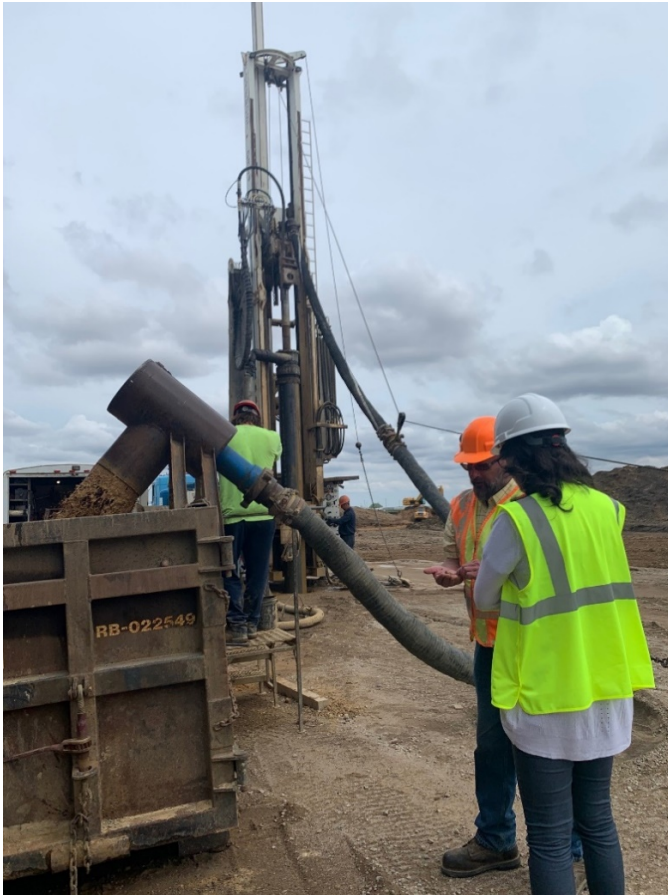
Figure 1. County Well Inspector examining cuttings from a non-community well to serve a population of over 25 at a new business.
