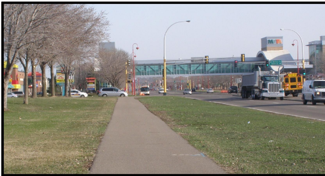
View of Cedar Avenue and the new pedestrian overpass north of 155 th Street/Whitney Drive.
