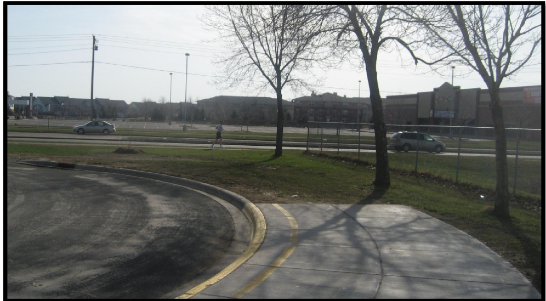
Gap between on-site sidewalk and the multi-use trail on Cedar Avenue.
