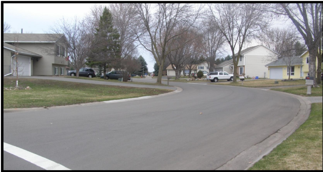
View of Dominica Court, looking north towards Diamond Path Elementary. There is currently no sidewalk on either side of the street.
