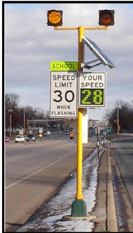
Example of a solar-powered driver feedback sign in a school speed zone in Anoka County.
