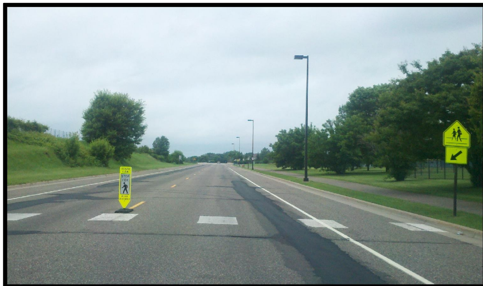
Existing in-street school crossing signing on Mendota Heights Road near St. Thomas Academy.
