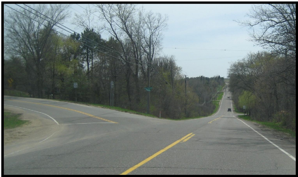
View of Delaware Avenue at Salem Church Road. The existing sidewalk and trail network on Mendota Heights Road, Huber Drive, and Copperfield Drive ends at Delaware Avenue.
