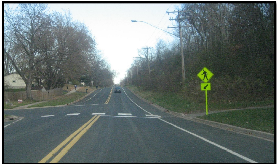
Area for proposed sidewalk connection on the south side of 130 th Street.
