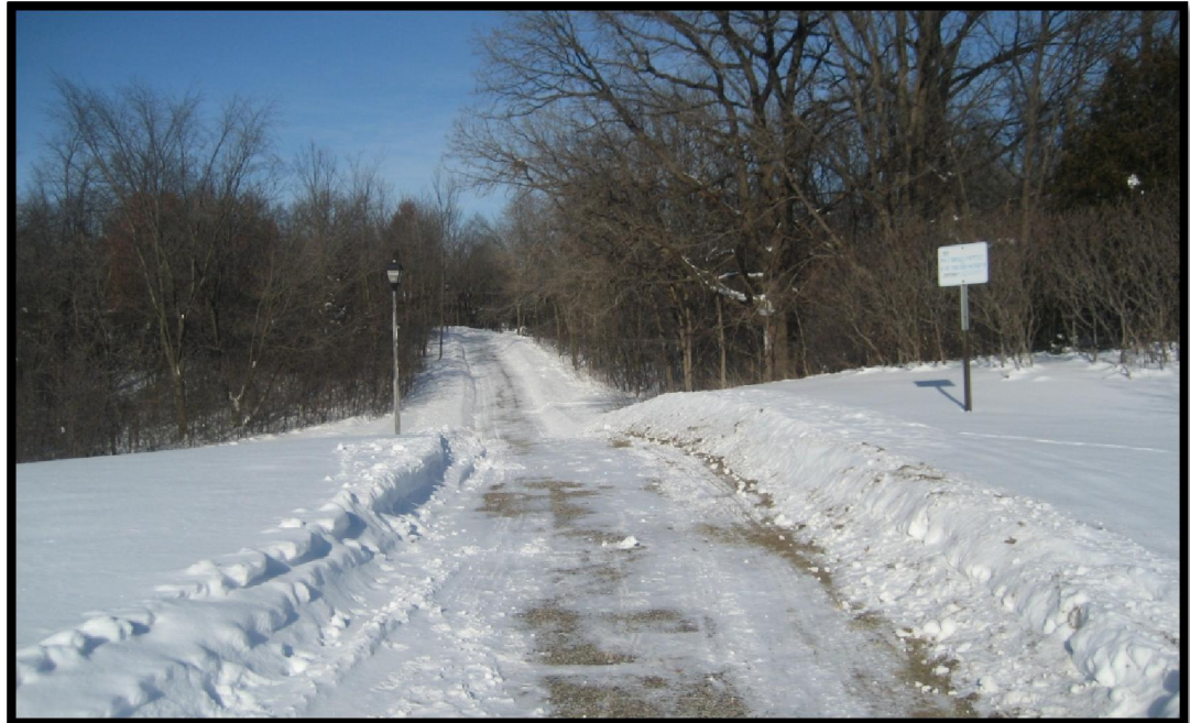
View of trail from Civic Center Parkway
