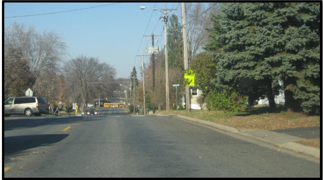
View of school crossing signing on northbound Pine Street at 11 th Street.
