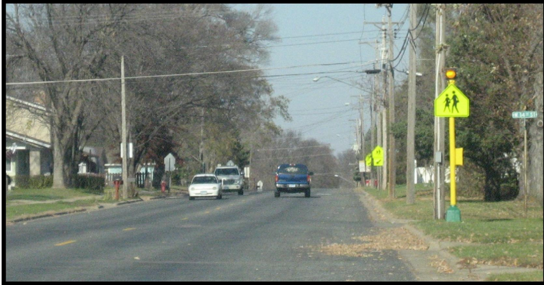
Advance warning flashers and school crossing signing on northbound Pine Street.
