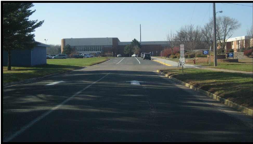
View of 11 th Street entering the middle school site. There are two one-way driving lanes, which expand to three lanes at the drop-off/pick-up area.
