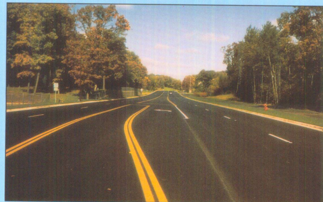
County Road 5 and Bike Trail in Burnsville.
