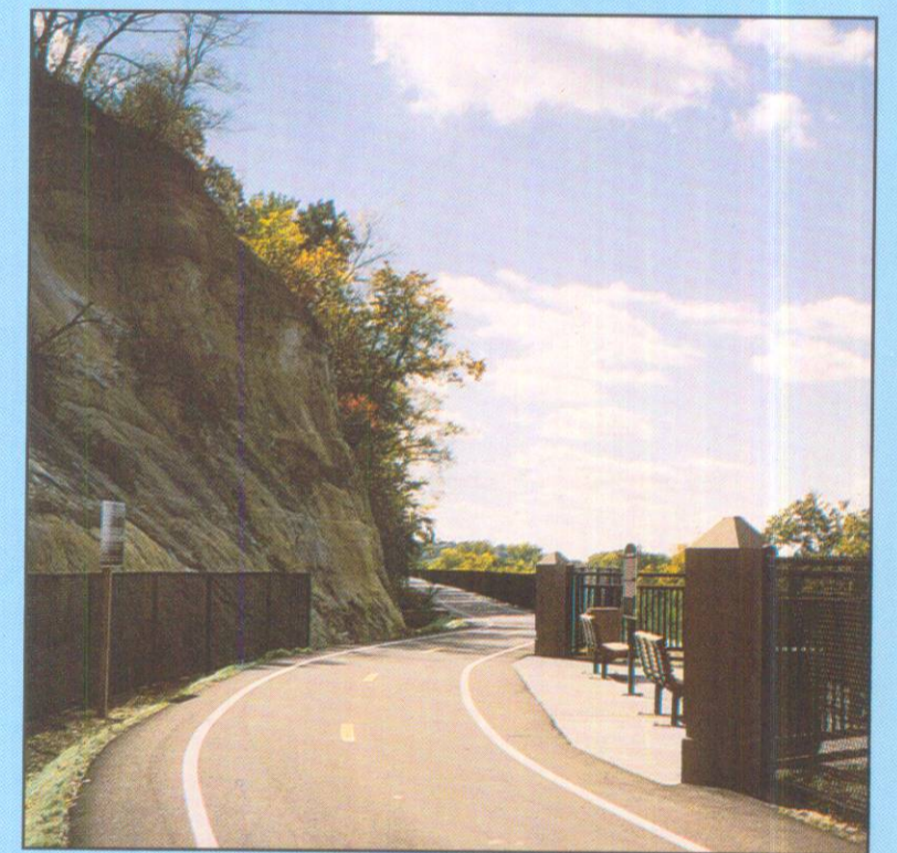
Big Rivers Regional Trail overlook when completed.
