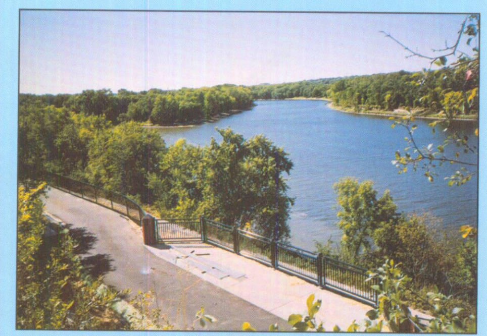
Big Rivers Regional Trail south overlook during construction.
