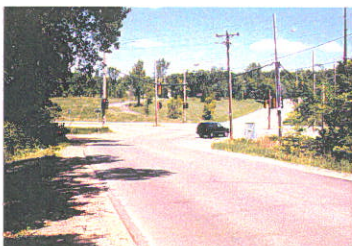
Existing Argenta Trail intersection. Note absence of right turn lane.
