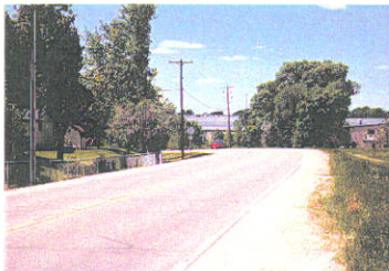
Argenta Trail - Winding/rolling alignment, limited sight distance.
