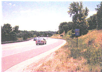
Substantial elevation difference at TH 3 results in cut sections that severely impact wetlands.
