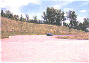
Existing CR 28/TH 3 intersection.
