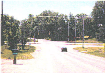
Existing Argenta Trail/TH 55 intersection.
