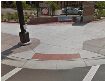
Example of a good or compliant pedestrian ramp
