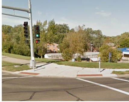
Example of a good or compliant traffic signal
