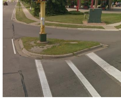
Example of a poor or non-compliant traffic signal
