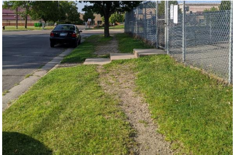
Figure 3-2: Example of Sidewalk/Trail Gap Where There is Demand for Walking to School
