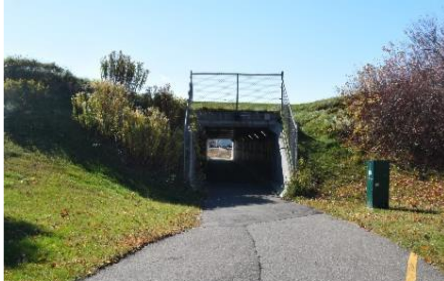
Existing tunnel under CR 46 (160 th Street) at East Lake Elementary
