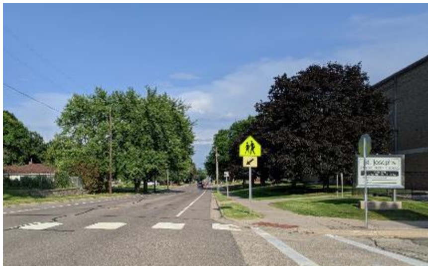
Existing school crossing on CR 4 (Butler Avenue) at Seminole Avenue
