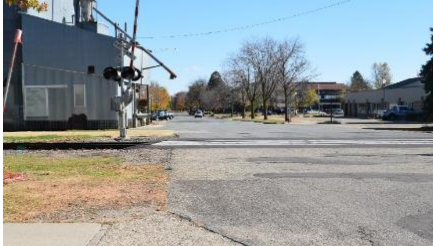
Existing sidewalk gap on Spruce Street at the Union Pacific Railroad
