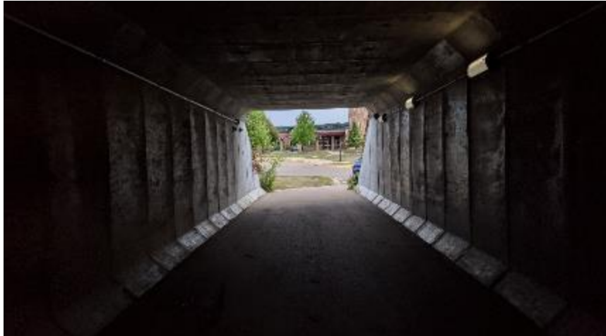
Existing tunnel under CR 64 (195 th Street) to Meadowview Elementary
