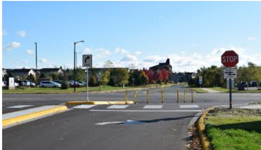
Revised school driveway at CR 9 (Dodd Boulevard) with exiting traffic restricted to right turns only
