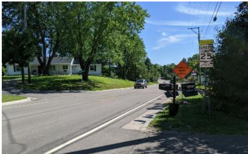
Existing school speed zone sign on TH 149 (Dodd Road)
