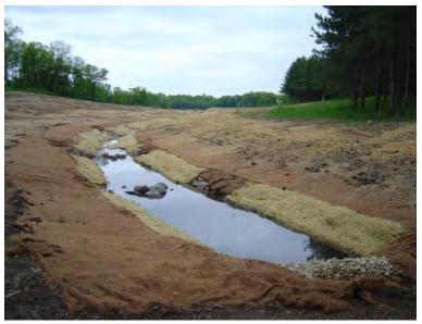
Marsh Lake Bio-swale Construction, 2008 Recommended in the 2006 Stormwater Management Plan, the bioswale cleanses water flowing from Marsh Lake to McDonough Lake.
