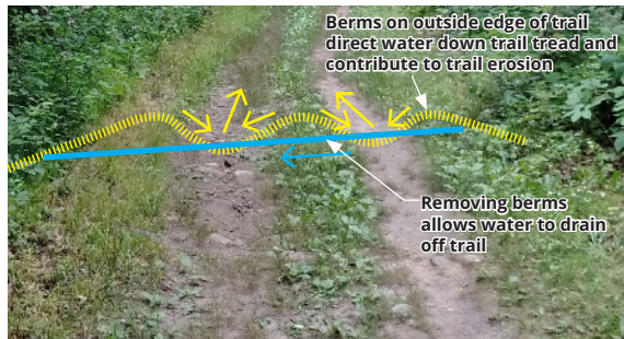
Example of trail in need of deberming at Lebanon Hills Regional Park the trail tread. The increased water volume and velocity will erode the trail.
