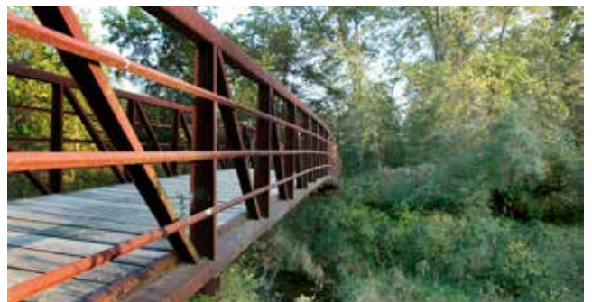
Bridge across Trout Brook
