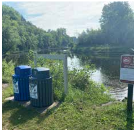
Eroded public water access site
