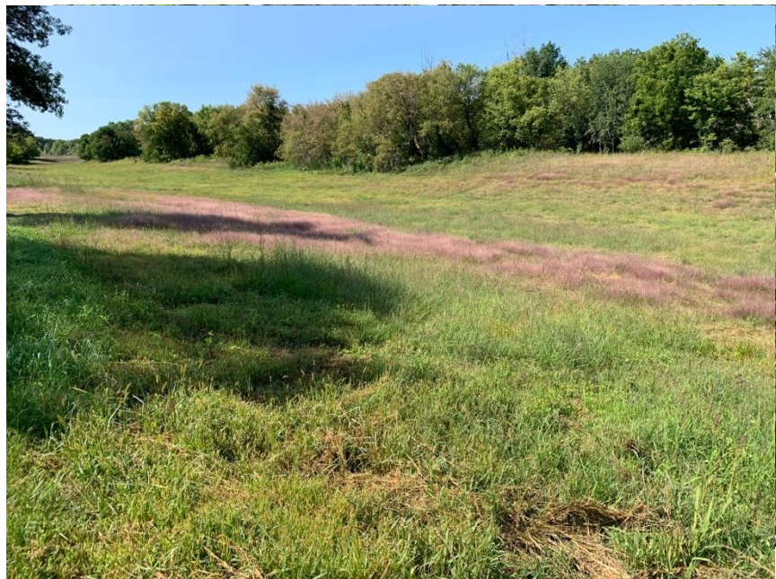
Photo 7. Spillway at Vermillion River Linear Park
