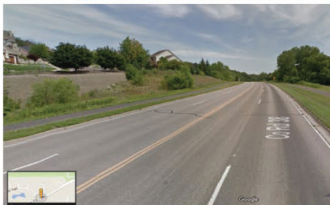
McAndrews Road Shoulder gap between Johnny Cake and Pilot Knob Trails on both sides of road
