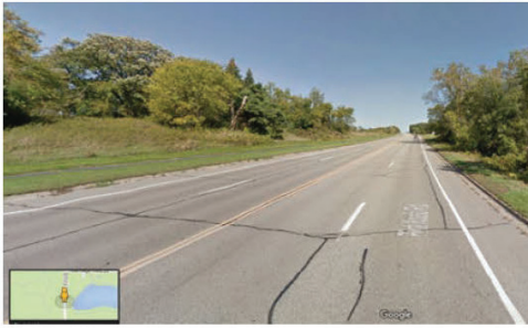
Pilot Knob Road 6' shoulder with curb and gutter Trail on west side of road only
