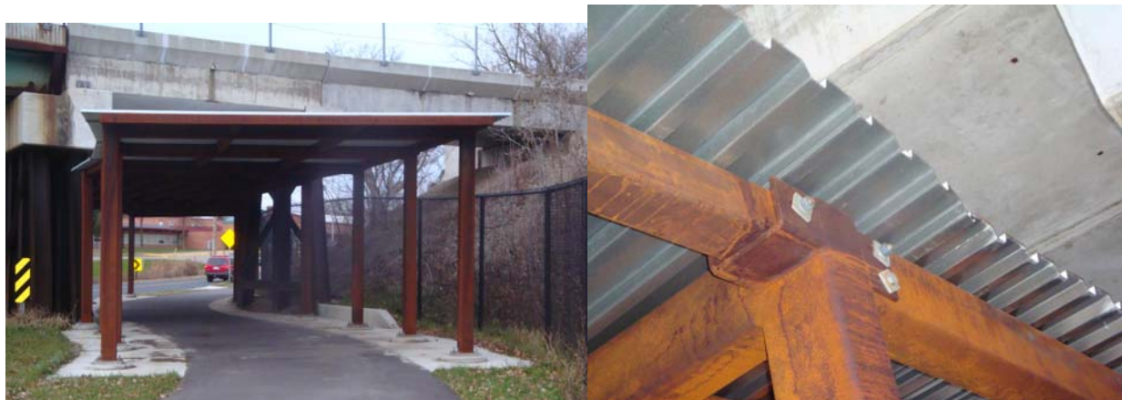
FIGURE 13 – Examples of Ballast Shield Structures
