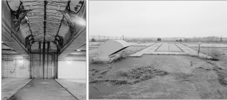
Nike Battery, inside the pit (left) and surface view with elevator doors closed (right). Photo: U.S. Library of Congress, Historic American Engineering Record, Andrew Baugnet
